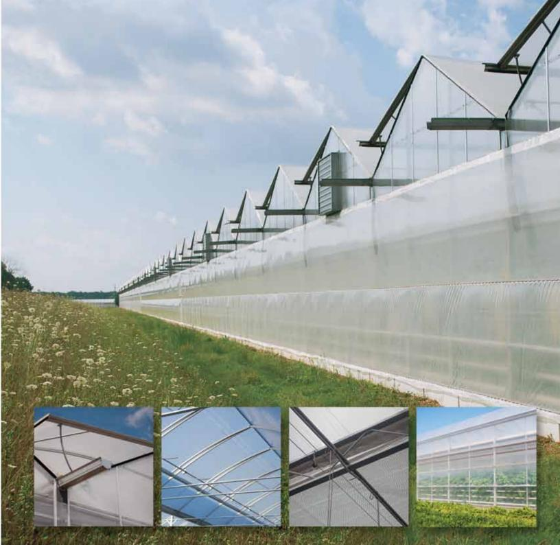
Continuous arch at calculated radius prevents poly wrinkles.
