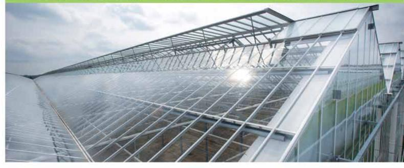
The Wide Span greenhouse offers a wider structure than the Venlo style greenhouse but is still built to the same strict standards. The roof components including the gutters are all aluminum and are available in various peak widths. Typically research centers, universities, and large garden centers find the wide span structure appealing for their various uses. The steel structure is hot dip galvanized and comes with the option of added powder coating to the colour of your choice.
